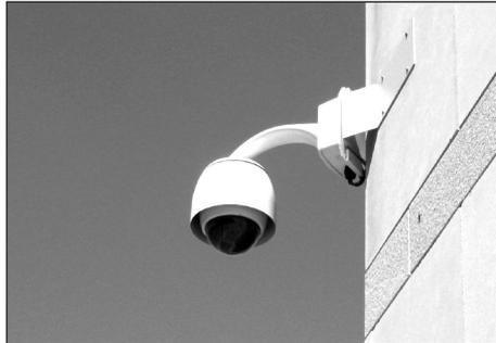
This semi-covert CCTV camera may have a crime prevention advantage over an overt system because offenders can never be sure in which direction that camera is facing.
