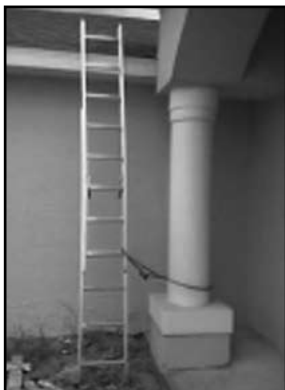
Example of target hardening of construction equipment.
